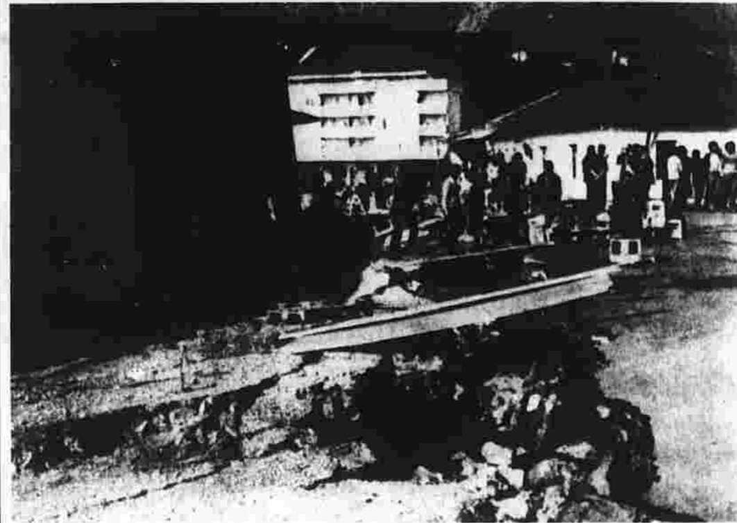
A huge crack divides the street in Bay of Notor, Yugoslavia, after an earthquake hit the Yugoslav southern Adriatic coast Sunday, killing at least 150 and injuring more than 600. (UPI photo)
